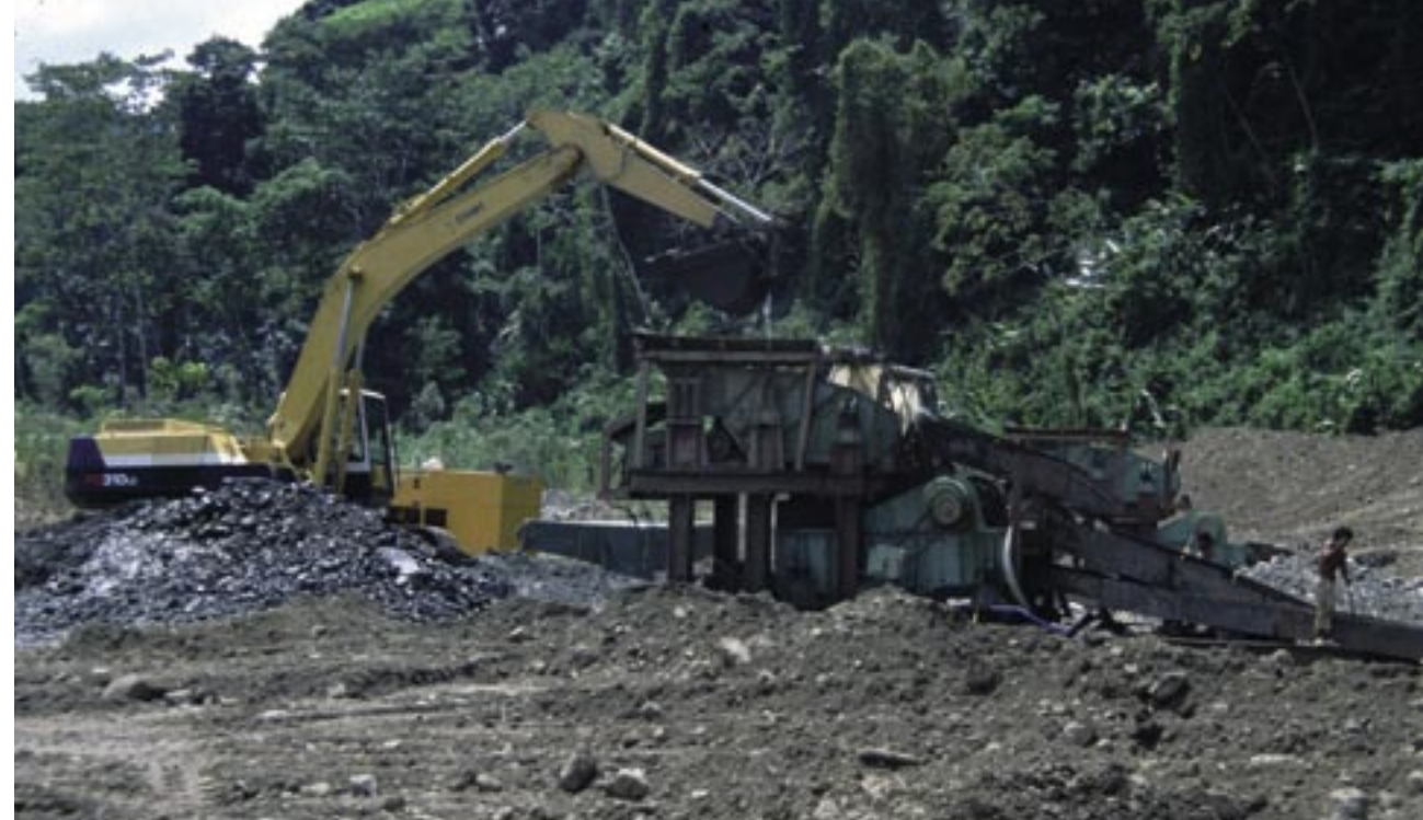
Clearing vegetation for development
